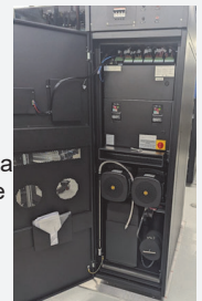
Figure 5: Steger Hall's first coolant distribution unit
