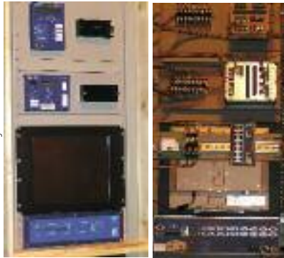
Left: New digital relays under construction for ECE. Right: Rear view showing the relay interconnection.
